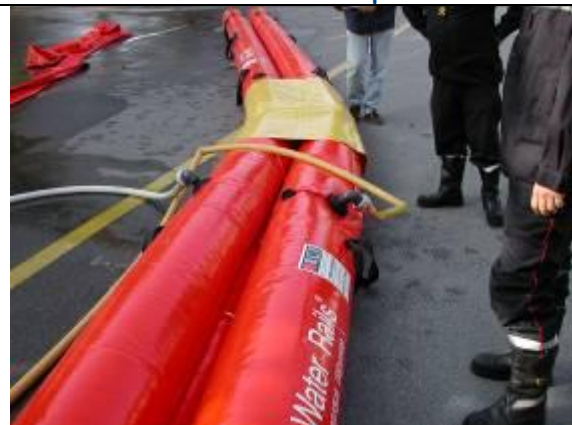
Joining the two lengths and filling the tubes with water
