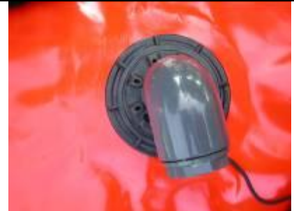
Setting up of the safety valve to control the level of the water
